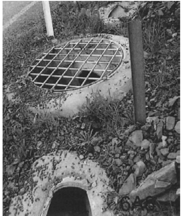
Pipe directing run-off from other farmland onto Ōhotu 6F1
