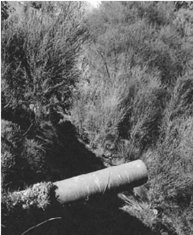
Culvert next to Parapara Road directing water onto Ōhotu 6F1
