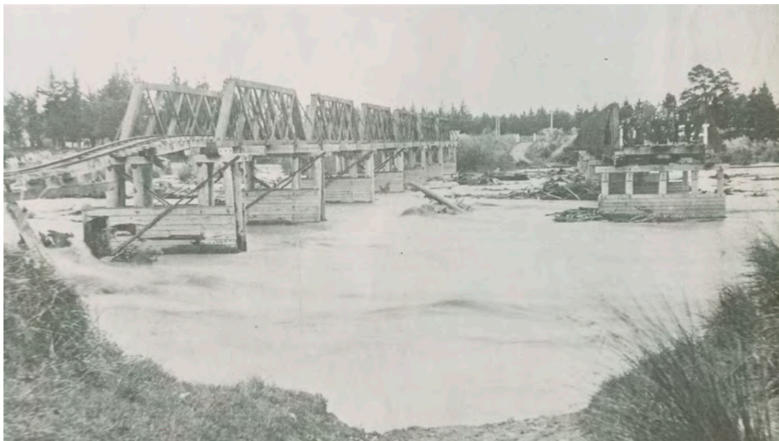
Figure 22: Damage to Aorangi Bridge on the Oroua River, after the 1897 flood. 557
