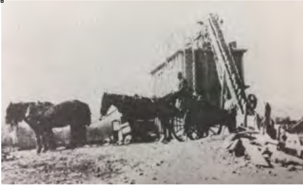
Figure 21: Gravel crusher at Waikanae a key facility in highway reconstruction. 543
