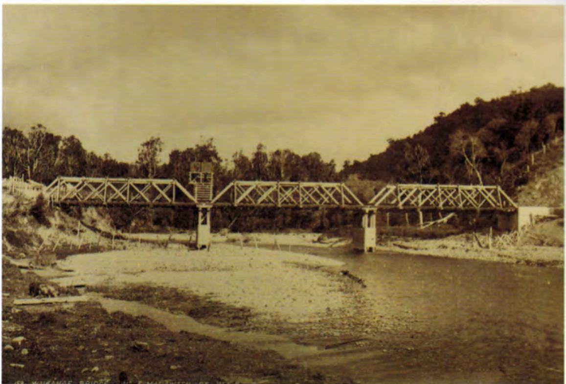
Figure 18: The first Waikanae River Bridge built between 1885 and 1888 for the Wellington and Manawatū Railway Company. 344
