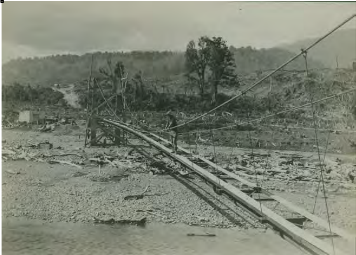
Figure 29: Ōhau River pipe-bridge in the course of construction. 756
