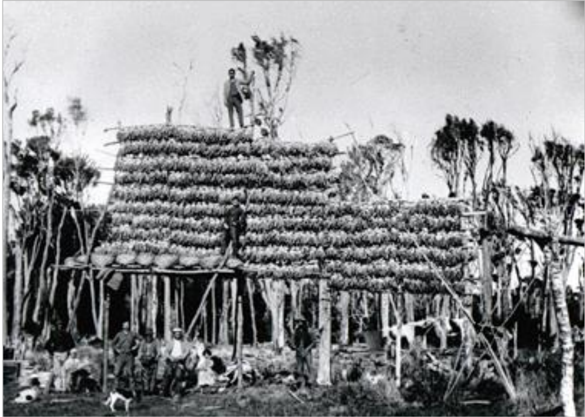
Image 28: Whare tupuna construction, Iwa te Kau mā Iwa
