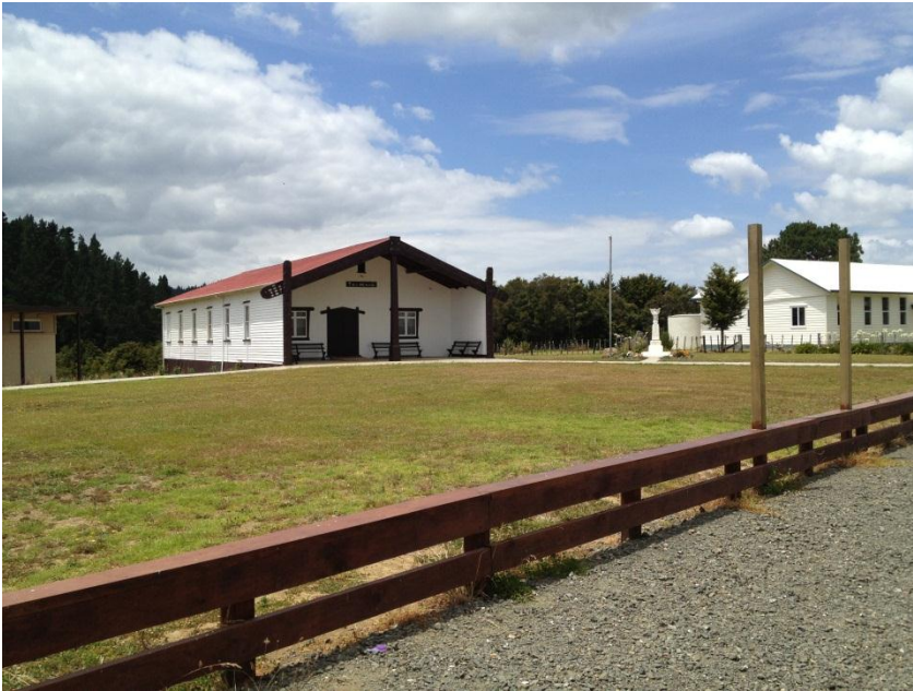
Figure 20: Tau Henare Marae and War Memorial, Pipiwai
