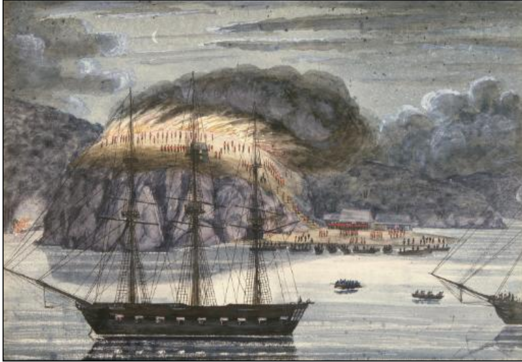
Figure 55: HMS North Star destroying Pōmare's pā, Ōtūihu, 29 April 1845
