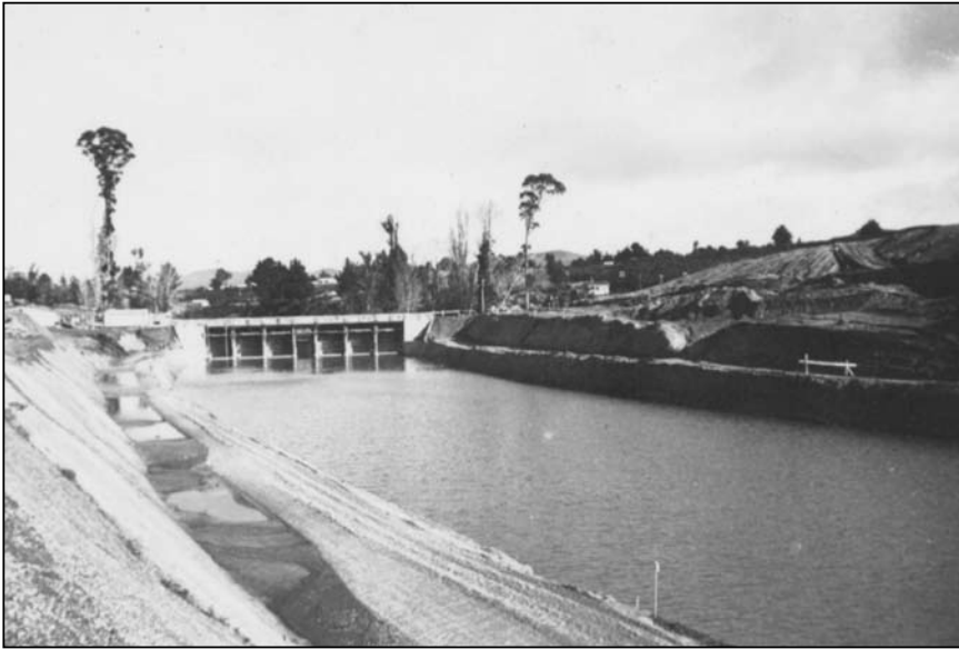
Control Gates under construction at Taupo, 1941
