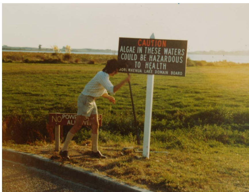
Image 5.2: Warning sign being erected at the lake, March 1976 1004
