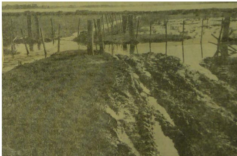
Image 5.1: Raw sewage flooding fields adjoining the lake, August 1964 936
