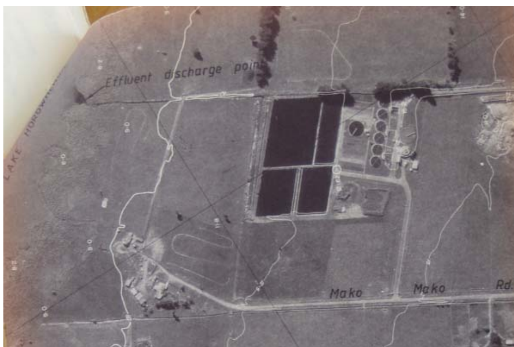
Image 5.5: Aerial view of the treatment plant, c. mid-1980s 1086
