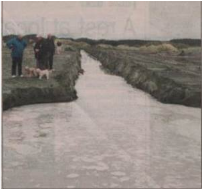
Figure 91: Newly dug channel at Hokio
